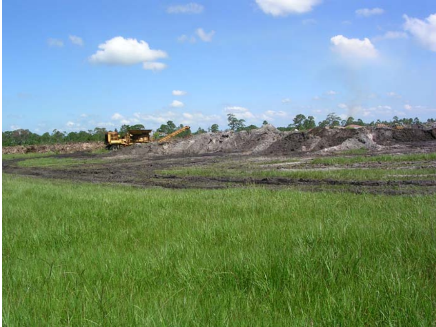
Photo 2.2. Looking West Toward Area Under Development, to the west of I-95.
