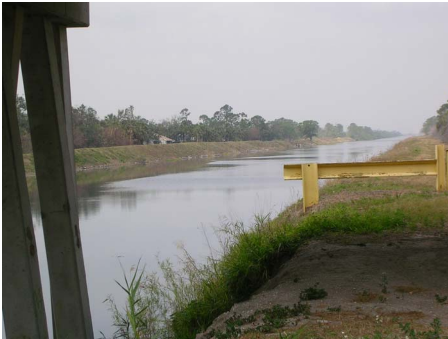
Photo 6.1. Looking East at the C-24 Canal from Beneath I-95.
